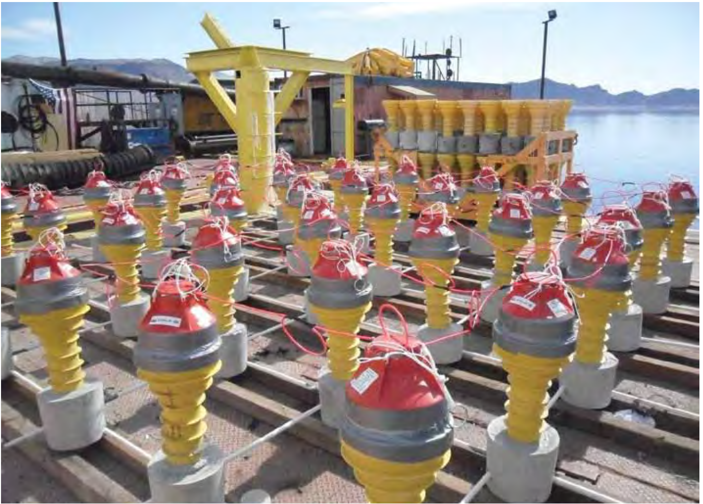
Figures 4 and 5. Charges on the barge, connected with detonating cord, with loops to absorb increase in distance when dropped in uneven lake bed. Net of detonating cord with redundant cross connections, ignited by a Pentolite booster. Plastic pipes kept charges standing at the right distance and to allow adjustment of the charge field to the uneven surface while keeping contact with the rock surface.
