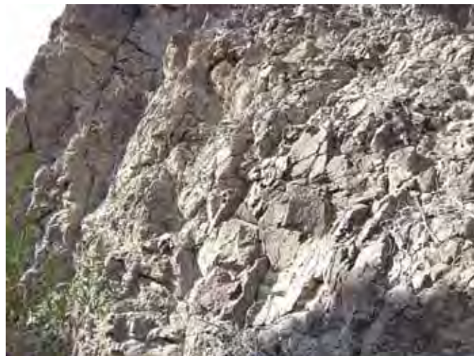
Figure 1. Callville, outcrop of the rock to be excavated.
