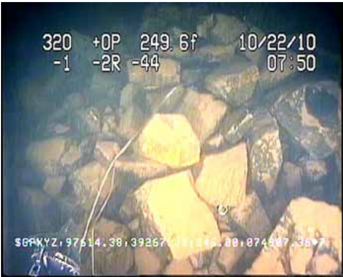
Figure 9. Muck pile underwater.
